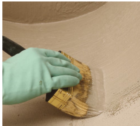
Waterproofing of details by brush
